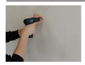
2. Drill holes, then mount brass clips using appropriate fixing system. Clips should be mounted along vertical axis
