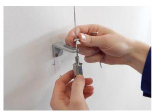
6. Install façade tightener to the bracket.
