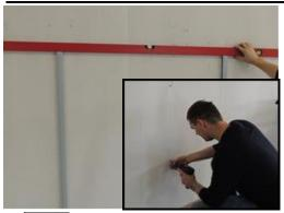
6. Set the level of upper edges of installed guide rails. Correct if necessary.
