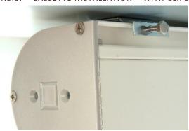
1. Put the cassette into the previously installed and leveled mounting clips. Then secure the cassette in clips by tightening the locking screw (use flat wrench).
