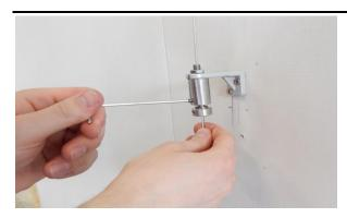
8. Loosen upper screw (locking movable part of the tightener). Stop when the movable part pulls out.
