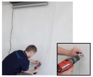
3. Mark places for cable bracket installation, then install the brackets.
