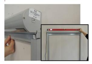
1. Put the cassette on guide rails, remember that the cassette has to be levelled horizontally.
