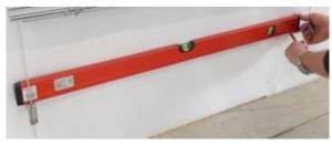
With a spirit level mark the installation place of the second cable guide bracket. Other actions perform analogically to the first bracket and guide.
