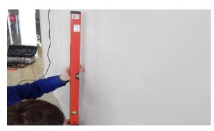
1. Check the vertical level of the cable. If necessary, correct by moving tightener in the bracket.
